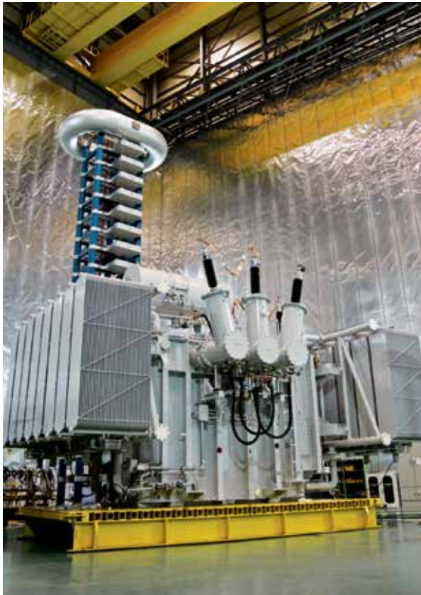
Shunt Reactor
