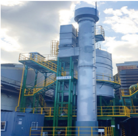
Replacement of an RTO (Regenerative Thermal Oxidizer)
