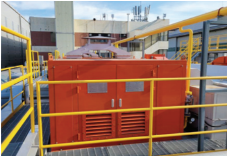
Replacement of a gas heater in the painting plant
