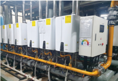
Installation of a cascade boiler
