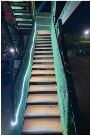
Installation of LED straps and upper flood lights on the access tower stairs
