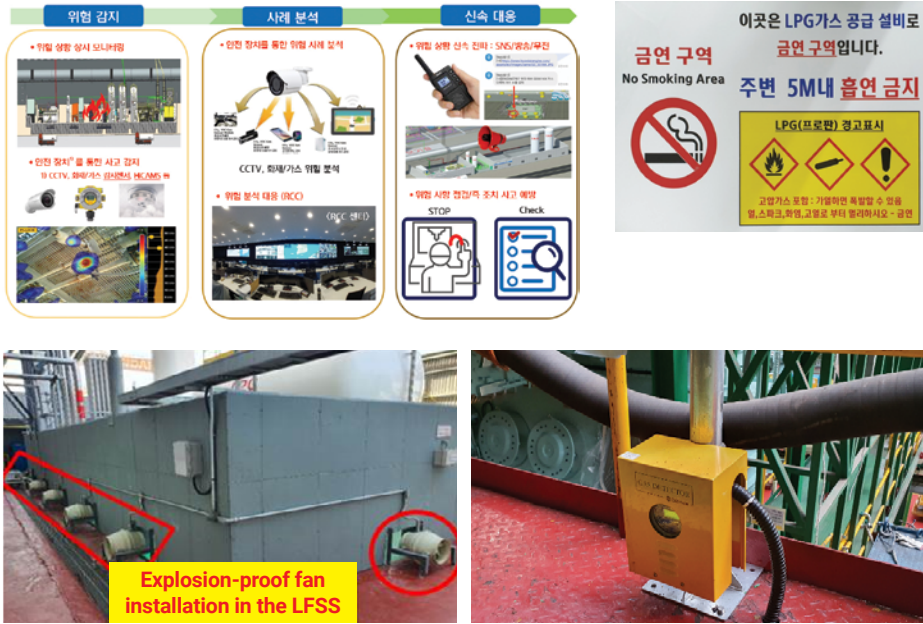
Gas Facility Ventilation Fan
