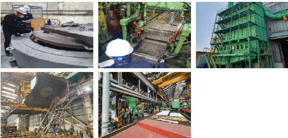
Measuring control velocity at hood, identifying duct damage, checking for filter/canvas damage, checking exhaust airflow
