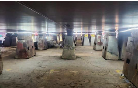
Installation of strap LED lighting on the dock floor
