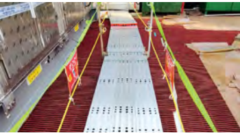
Scaffold reinforcement and safe passage route setting
