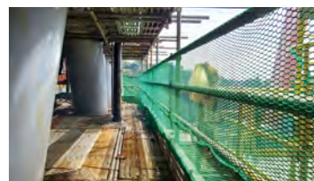
Falling object prevention net installation
