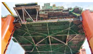
Falling prevention net installation
