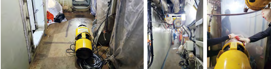
Jet fan installation to improve internal ventilation for surface vessels
